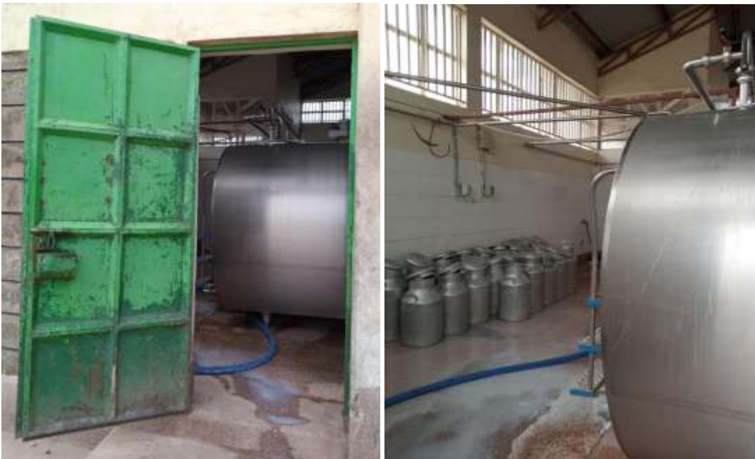
Photo: Chilling Room
