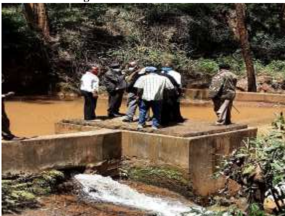
Photo 3: Inspection chamber for existing gravity main line along the road
