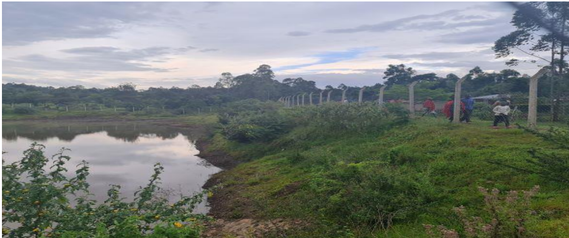
Plate 2: Soil erosion on the embankment
