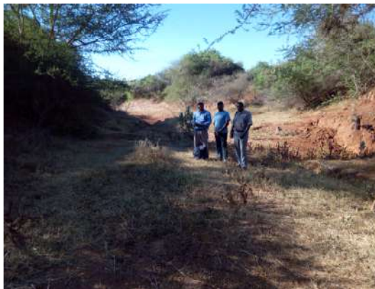
Part of the Mkuru water way at the point of the dam construction site. The back ground leads the water downstream into ranch land and Tsavo National Park.
