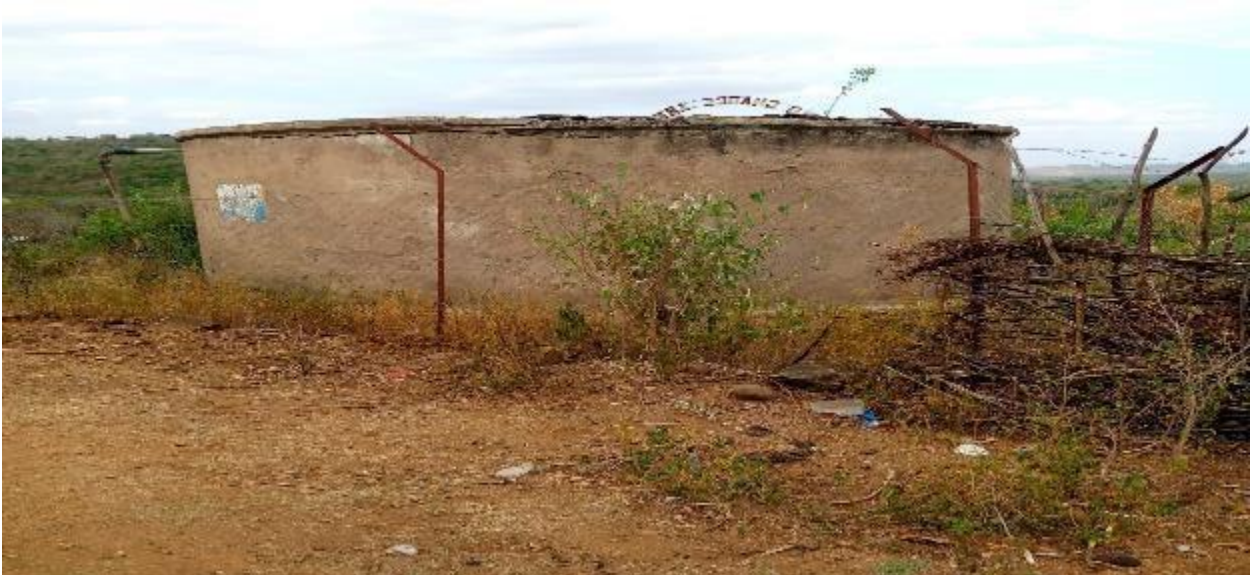
Photo 6: Tank to be rehabilitated
