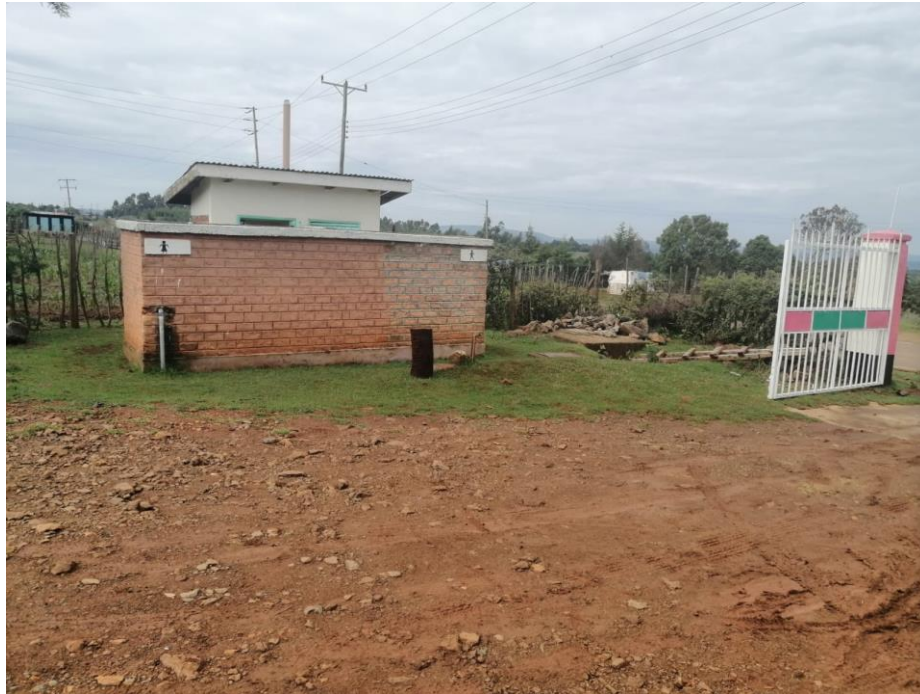
Figure 6.7. Existing pit latrine on site
