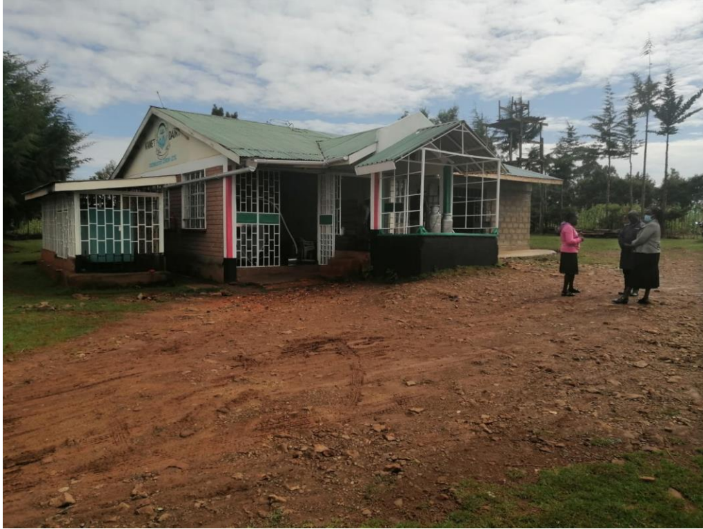
Figure 2.3: The facility has no washing and drying stand for milk cans
