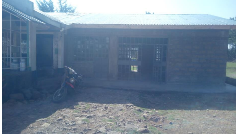
Photo 1: Building to house yoghurt processing activity
