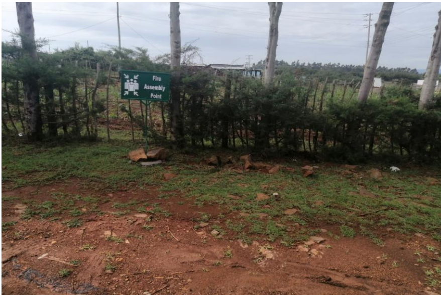
Figure 3.8: A solid fence e.g. brick wall or iron sheet fence should be constructed to replace this fence
