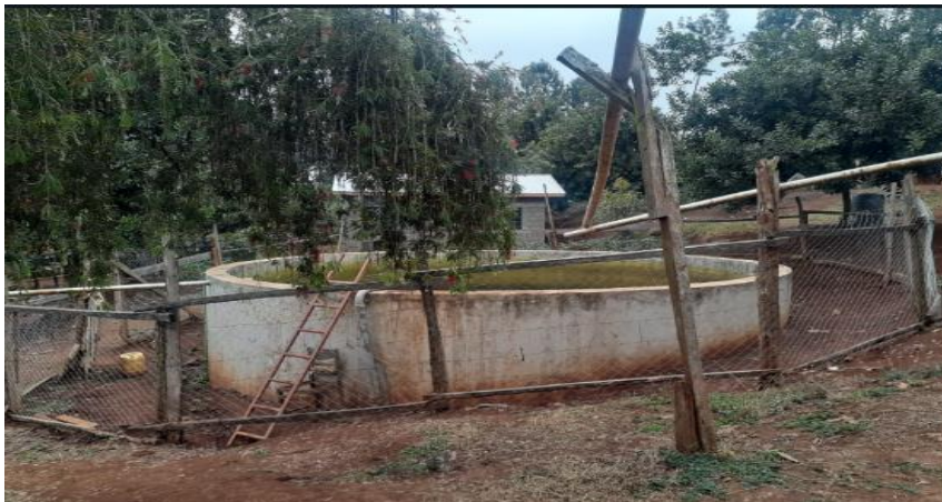
Figure 2 Roof harvesting at the factory with a storage tank
