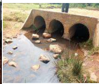
Existing spill-way area
