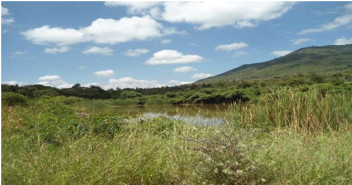
Plate 3: A photo showing over-vegetated area surrounding the earth dam
