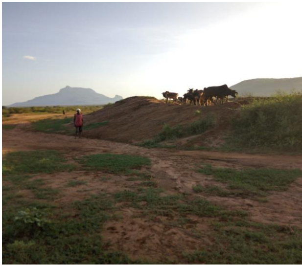
Livestock scaling the dilapidated pan walls to access water
