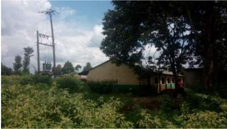
Figure 3: View of the electricity transformer near the proposed project site.
